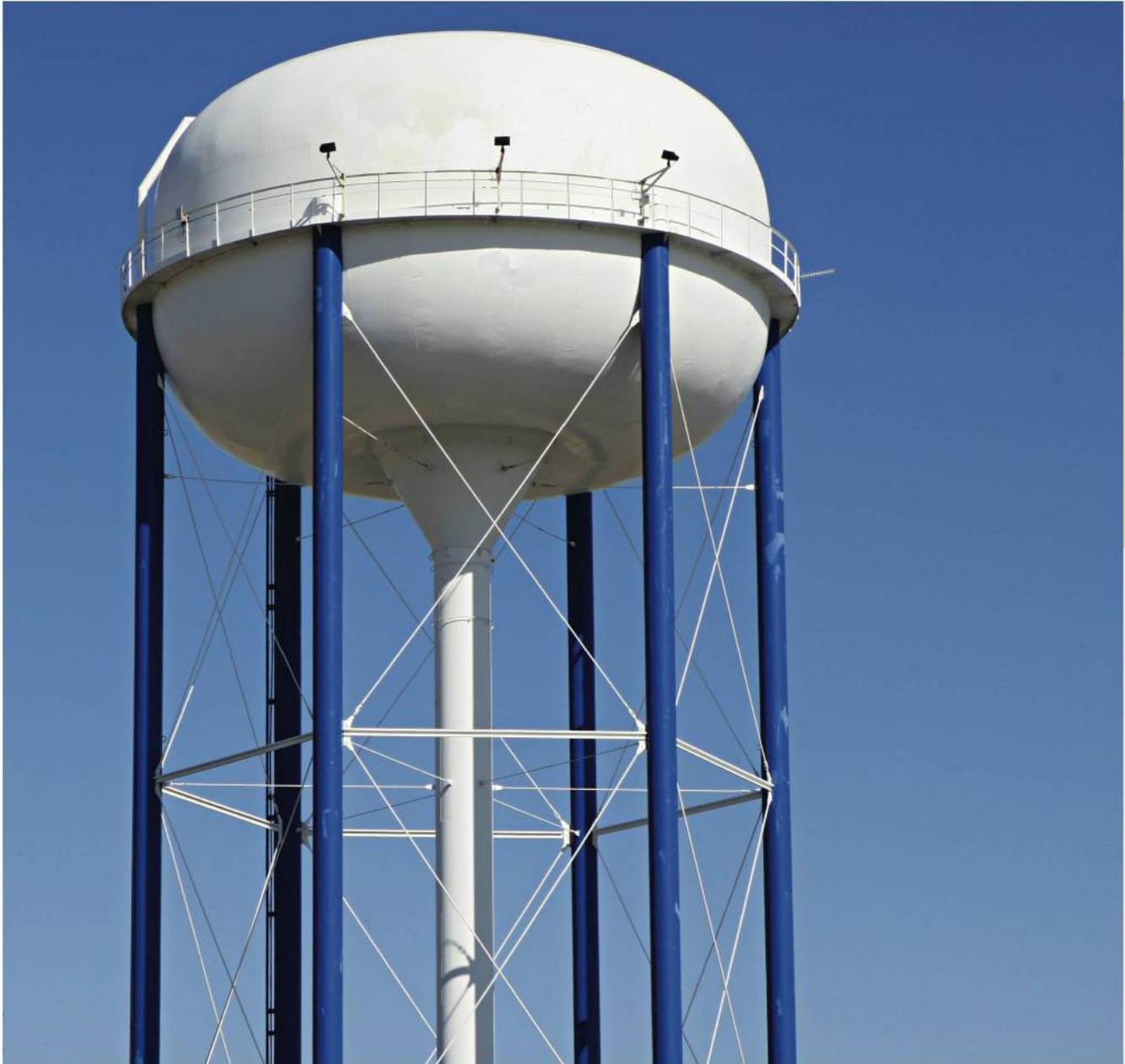
The columns of this water tank are braced at their length in order to reduce their chance of buckling.
